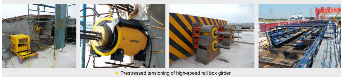
▲ Prestressed tensioning of high-speed rail box girder.
